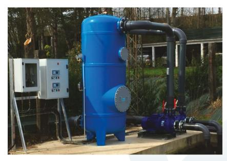
Outlet oxygen concentration: 700% of the saturation. Efficiency > 90%.
