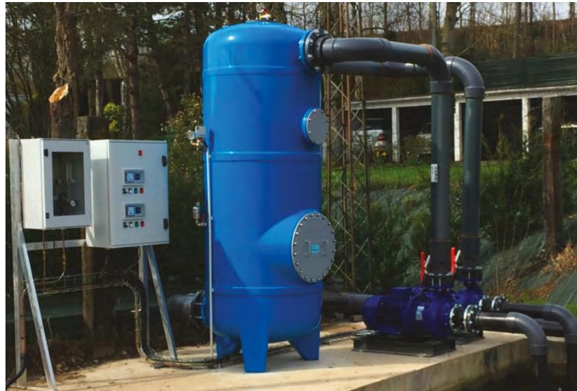
**Outlet oxygen concentration : 700% of the saturation. Efficiency > 90%.**
